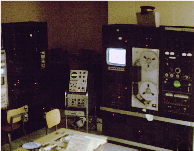
Success! No smoke, fires or tripped breakers!
